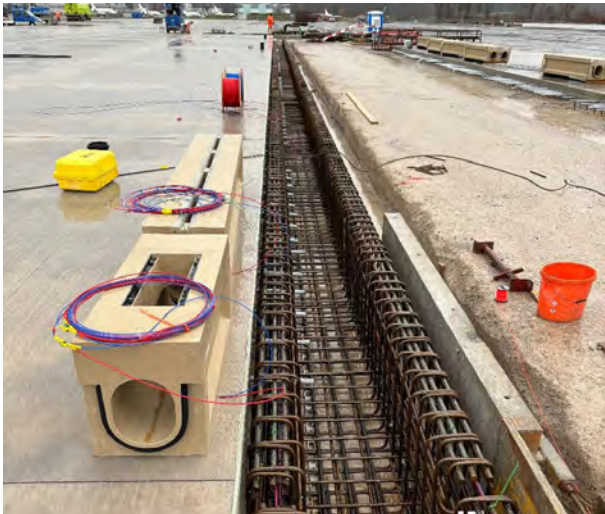
Installation of distributed sensors in the Zürich Airport. Quelle: Antonio Salazar
