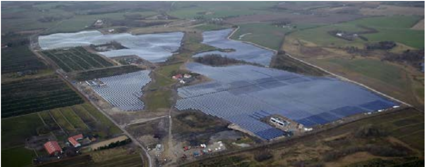
World's largest collector field in Silkeborg DK with 157'000 m 2 of flat plate collectors generating 20 % of the district heating energy demand.
