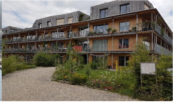
Figure 28: View of building B with roofs 1 to 3.
