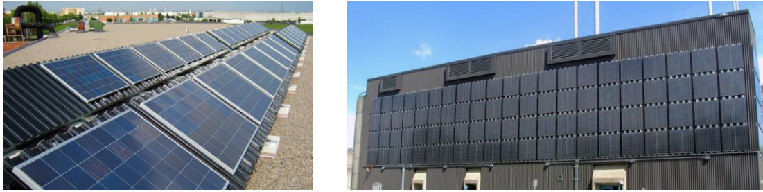
Figure 11: Air PVT systems “SolarDuct PV/T®” (left) and “SolarWall PV/T®” (right) from Conserval Engineering. Photos: Conserval Engineering.
