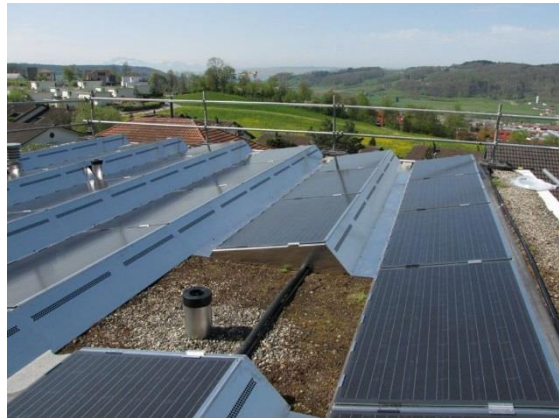
Figure 25: View of the PVT system on the roof of the single-family house in Wettswil.
