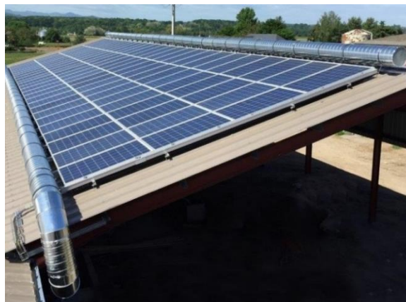
Figure 24: Air PVT system for drying grass in the French province of Béarn. Product from Cogen'air (BASE). Source: BASE Innovation.
