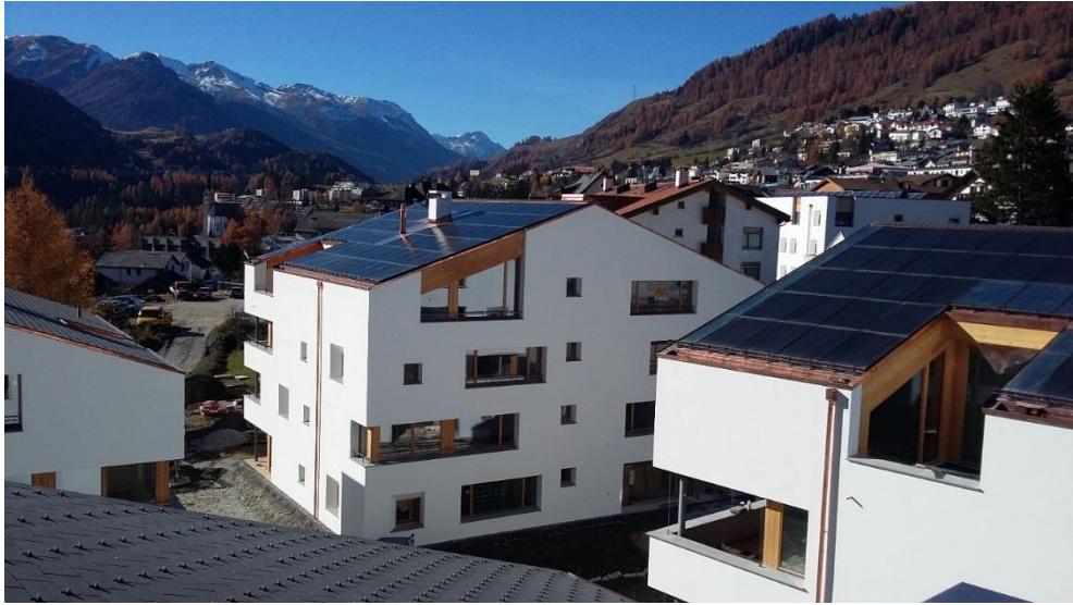
Figure 40: Sothà complex in Scuol. View of building B (PVT) in the middle; on the right, building D with PV system. This building is not structurally identical to the others and therefore does not form an integral part of this pilot and demonstration project.
