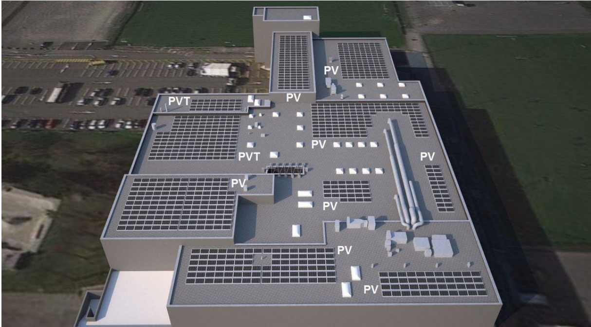
Figure 38: Aerial view of linth-arena, 3D model produced by the Solar Technology Team at the Zurich University of Applied Sciences, Wädenswil. Source: Zurich University of Applied Sciences, Wädenswil. The image shows the various PV fields (total surface area, 1,146 m 2 ; 180 kWp electricity) and the PVT field (292 m 2 ; 48 kWp electricity).
