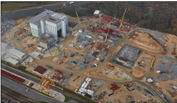
Hitachi Zosen Inova Construction Site Hitachi Zosen Inova AG (2019)
