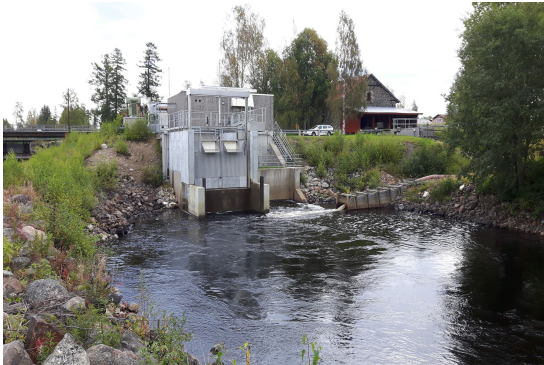
Hydro power plant in Robertsforts, Sweden, with two turbine outlets (centre) and a fish way combined with an attraction water pipe (right).
