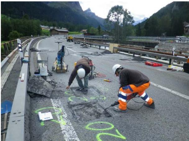
**Figure 4: Probing on bridge**
