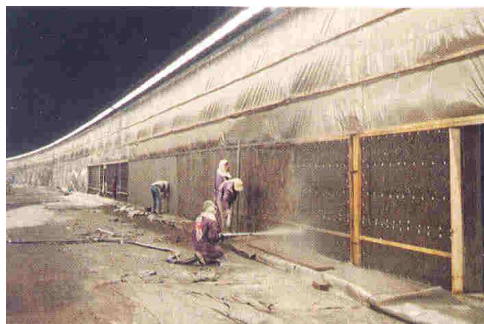
Fig 12: Gotthard tunnel entrance
