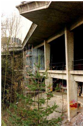
Fig 8: Supports at the station square
