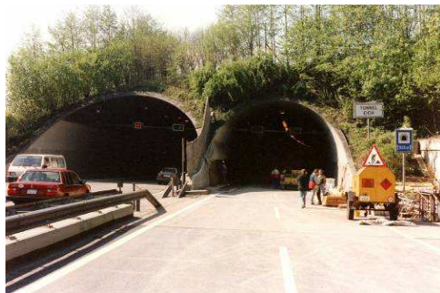
Fig 11: Eich tunnel near Eich
