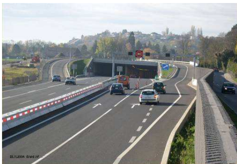
Fig 15: A5 highway tunnel
