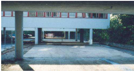
Fig 13: Parking garage in Baden
