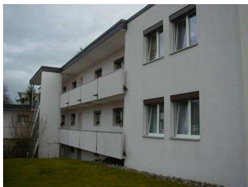
Fig 21: Apartment building in Adliswil
