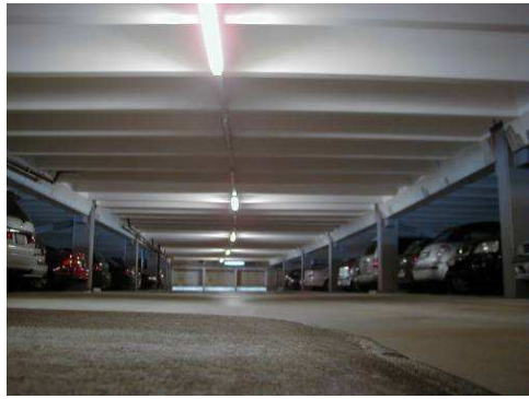
Fig 22: Airport parking garage
