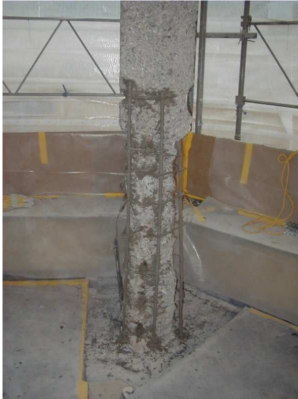
Fig. 1: Support during the repair
