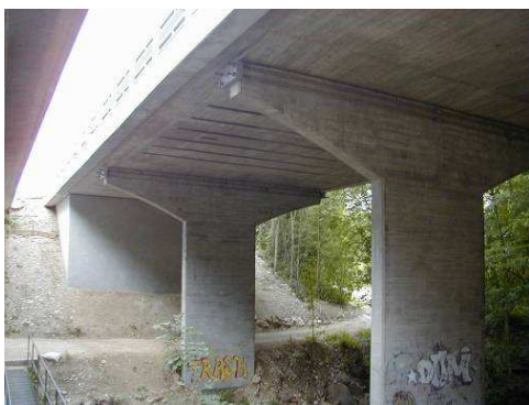
Fig 17: Siggern bridge near Attiswil
